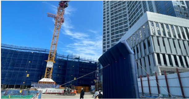
Installation of sound insulation wall
