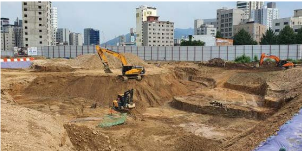
Excavation of contaminated soil
